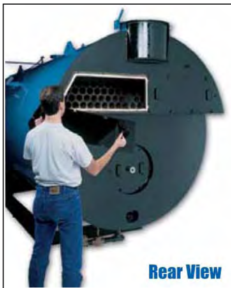
Securing the doors on a Burnham wet back boiler requires no specialized skills or expensive repair materials.
